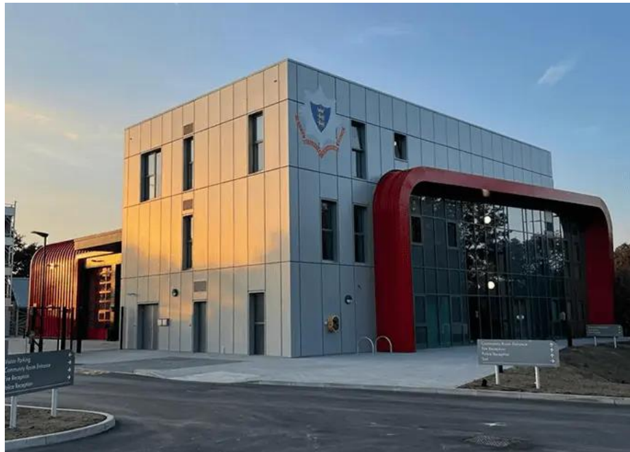
Figure 1 – Theale Tri-Service Fire Station (Completed 2021).
