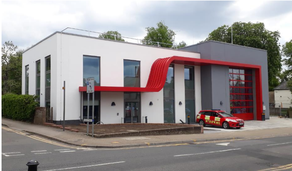
Figure 5 – Crowthorne Tri-Service Community Station (completed 2020).
