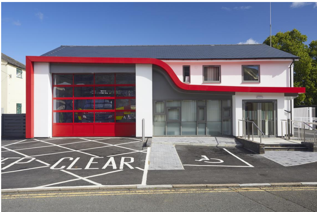
Figure 4 – Hungerford Tri-Service Community Station (completed 2017).
